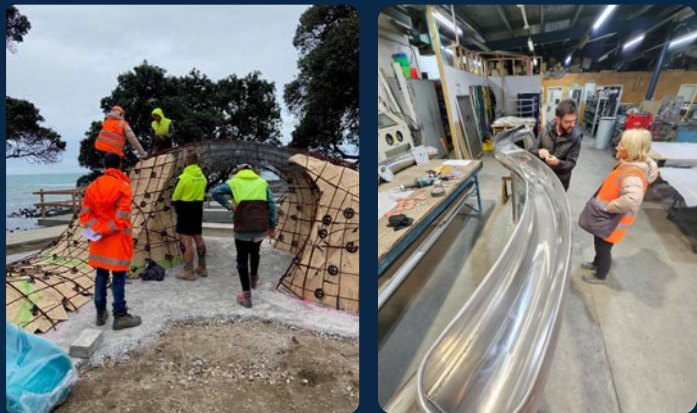
Quality Assurance Playground Safety Auditor inspecting waterplay and sensory zone climbing features as they were developed
