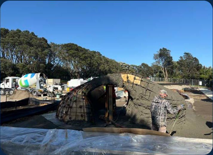
Sensory Play Zone construction
