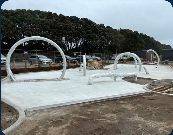
Water Play Zone construction
