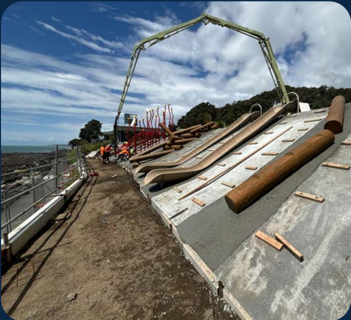
Hill Play Zone construction
